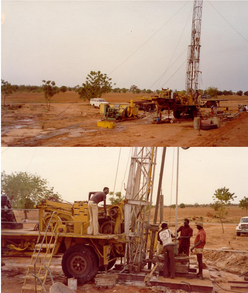
FIG. 6-02 BALLERINI PR1 Rig at work in Sokoto State of Nigeria, 1980
