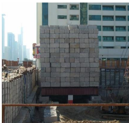
Figure 4. Loading test using kentledge Dubai (Fugro).
