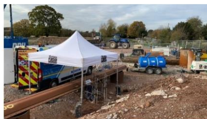
Figure 6. Bi-directional loading test underway (Fugro).
