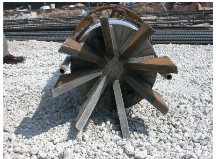
Figure 3: arrangement for connection to the reinforcing cage.
