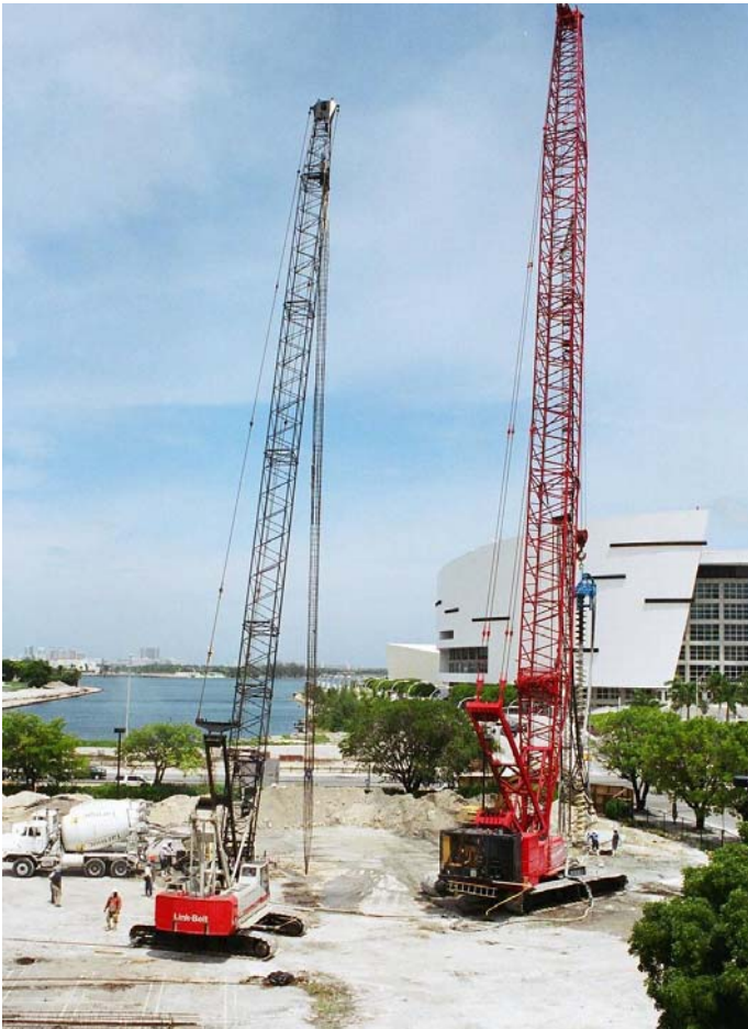
Figure 2: 50m cage ready for insertion into pile.
