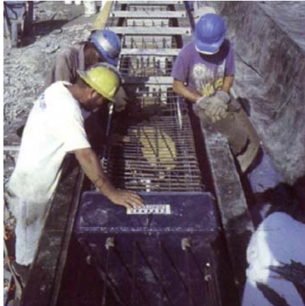
Installing an O-cell into a precast pile
