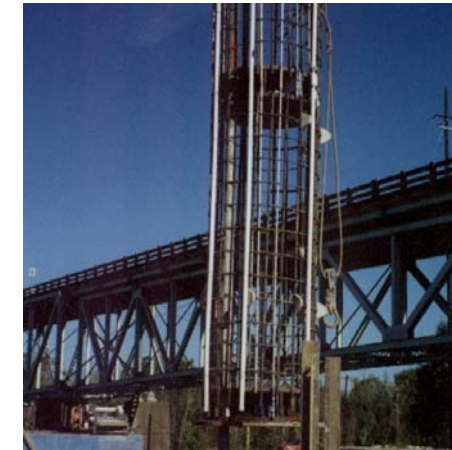
Multilevel O-cell assembly
