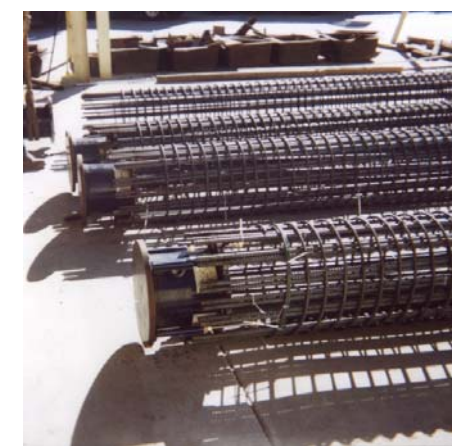
Testing multiple test piles
