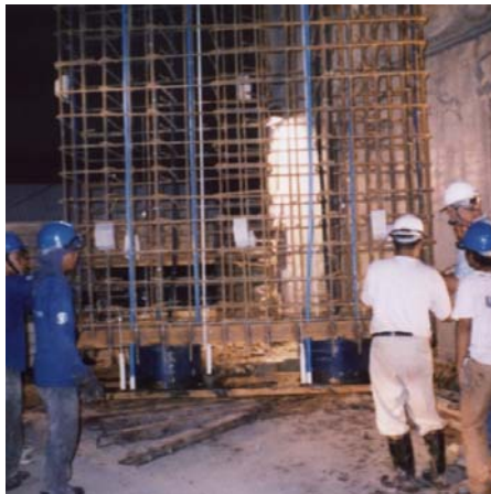
Installation of O-Cells into a barrette
