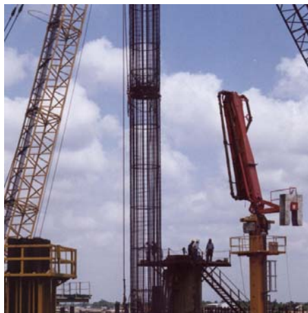
Test shafts/piles from 4.5-107 m have been successfully installed. Precast piles as long as 40 m have been driven and tested with the O-cell.
