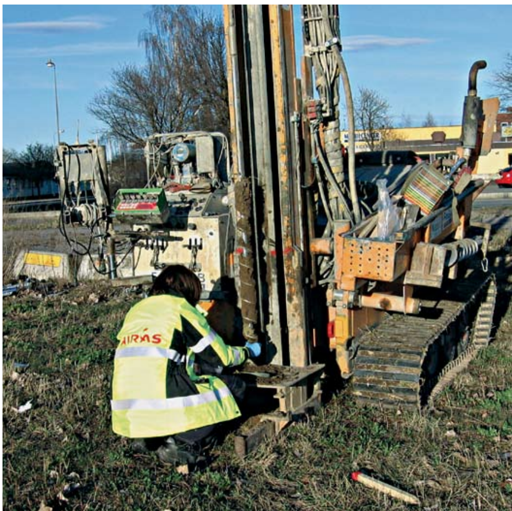
Taking tests in the field (Butängen, Norrköping, Sweden)
