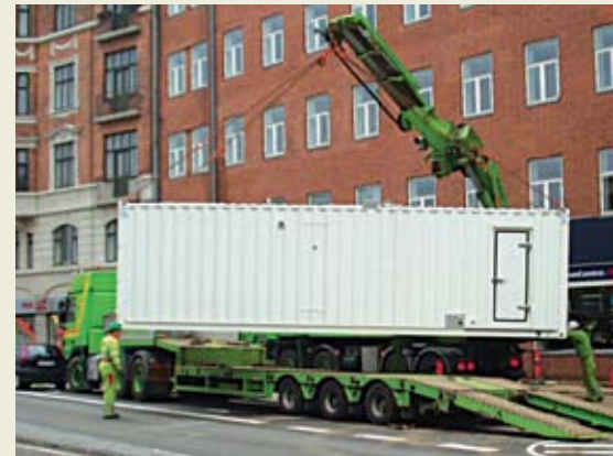
Setting up an on-site bioreactor in the city of Copenhagen (Denmark)
