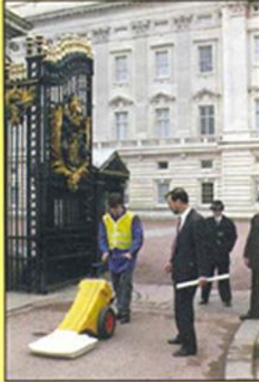
EMRAD were recently asked to locate the gas main running near to Buckingham Palace.
